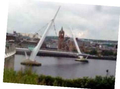
Editor's Note: Isn't it amazing what combined weight can do – It's going to cost a fortune to repair those uprights!!
